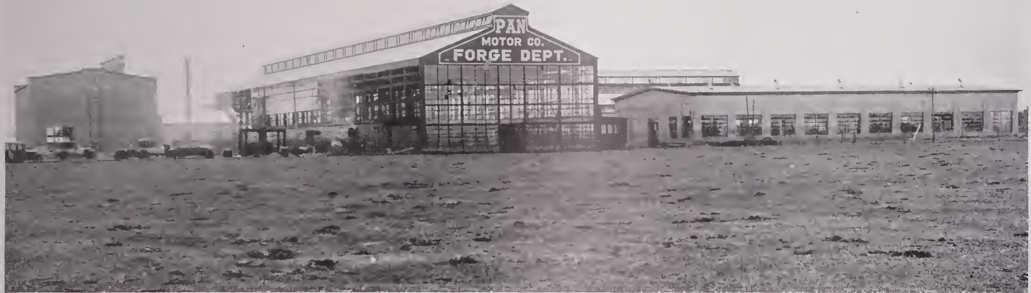
THE DROP FORGE PLANT FROM THE NORTH
